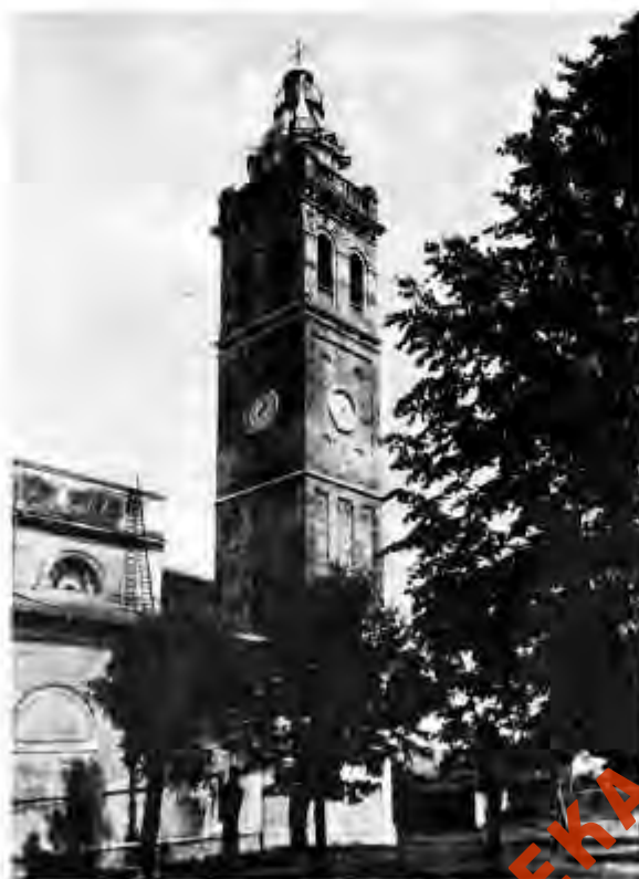
Bell tower of the Cathedral of Shkodra. The Cathedral built in 1858 was the largest church building in Albania. The bell tower was demolished in the fall of 1967, following the violent attack against religion. It is now a sports arena.
